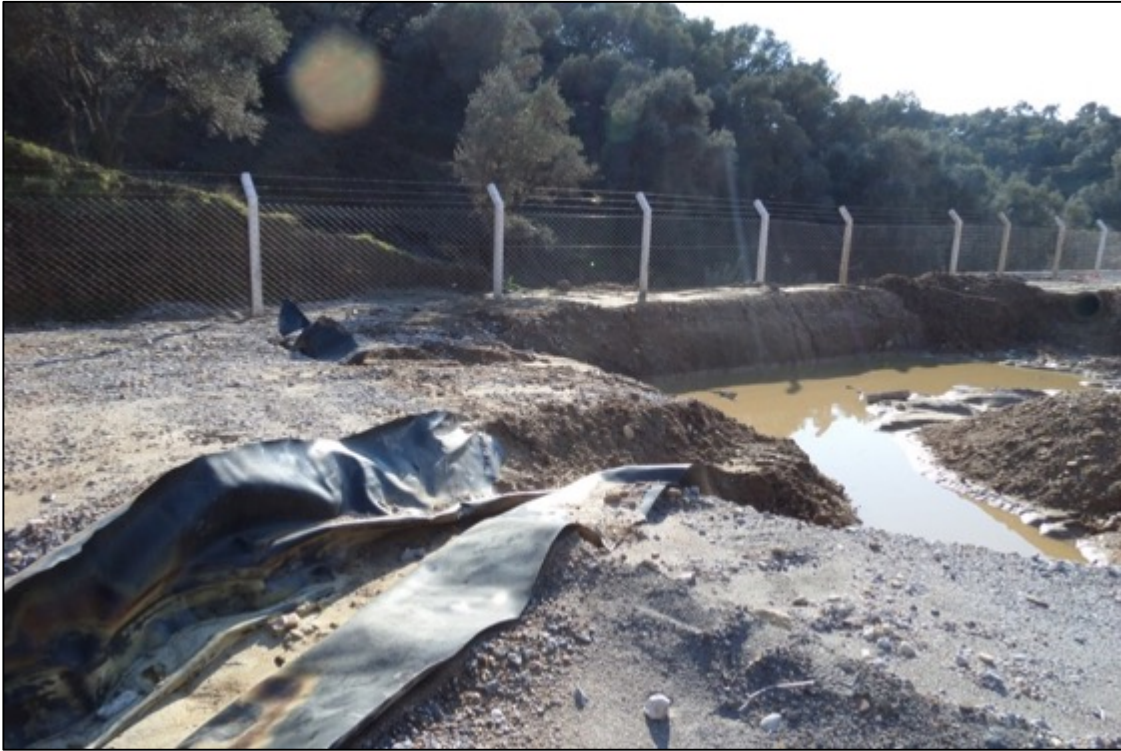
Photo 7-1. Mud Pits Lined with Geomembrane
