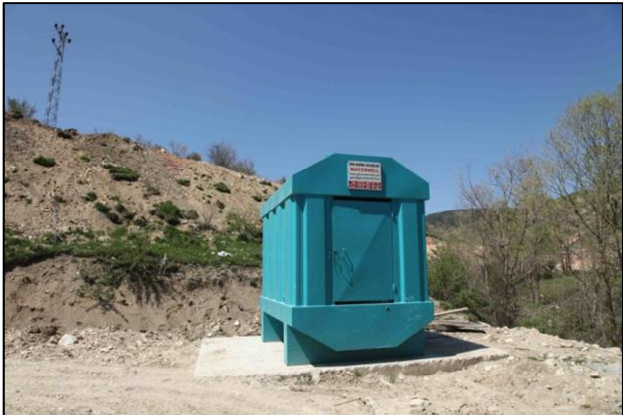
Photograph-7. The Biological Package Treatment Unit
