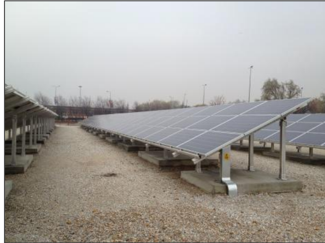
Figure 4-3 PV Panels and Holders
