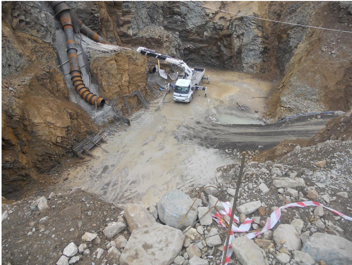
Annex 7.3: Power Plant Area (Before Construction)
