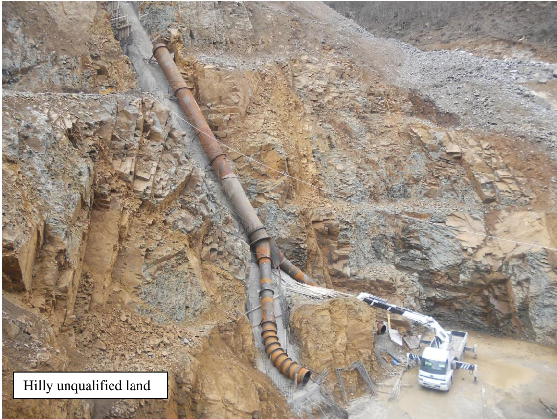
Annex 7.2: Penstock (During Construction)
