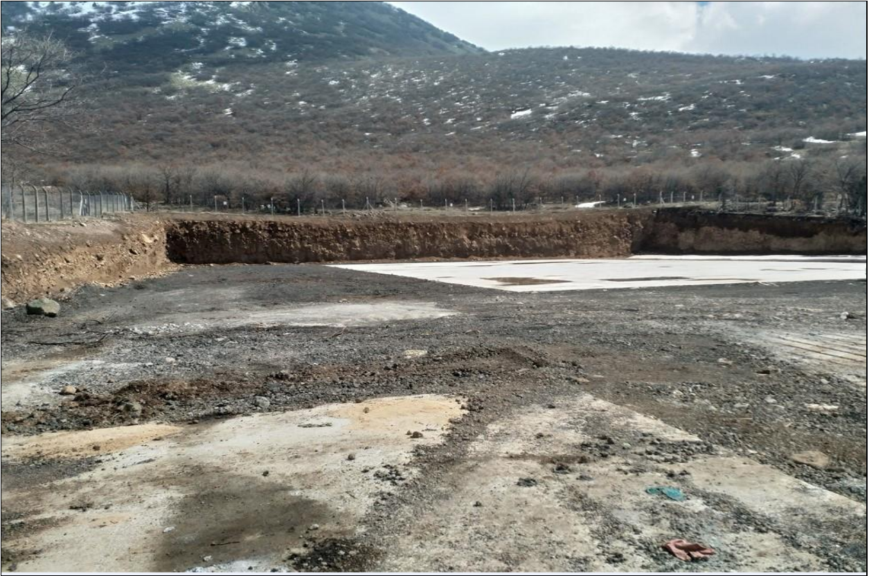
Figure 22. Drilling Location Photo (1) (Çömlekçi Project)
