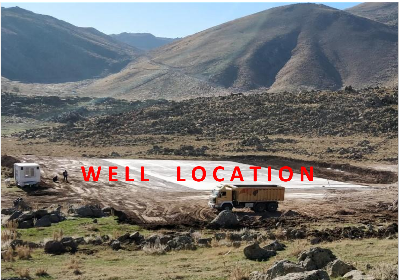
Figure 21. Drilling Location Photo (4) (Kitreli Project)
