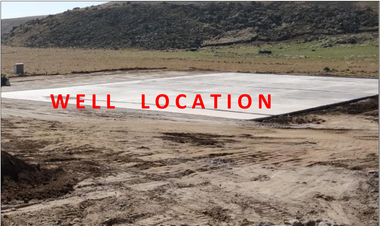
Figure 20. Drilling Location Photo (3) (Kitreli Project)
