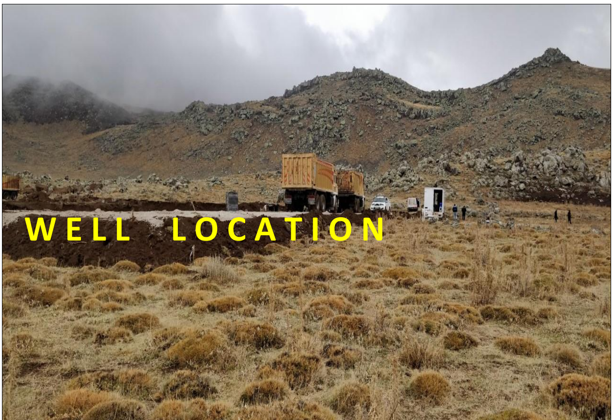
Figure 19. Drilling Location Photo (2) (Kitreli Project)
