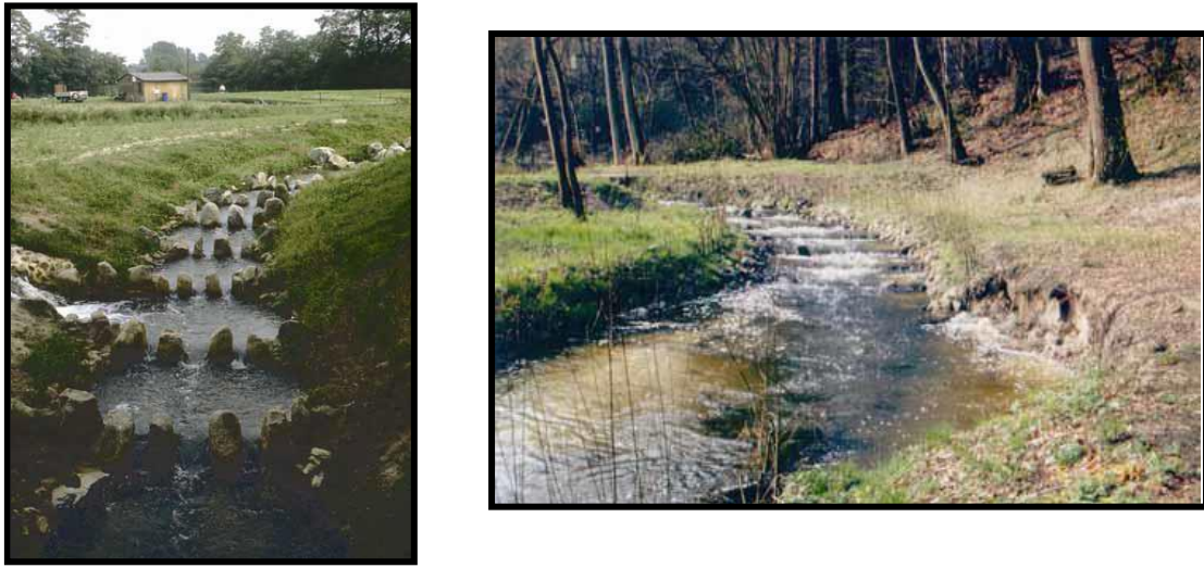
Figure 5.2.3.3. Bypass Channels of Varrel Bake Stream and Stöbber River (SHW, 2009)
