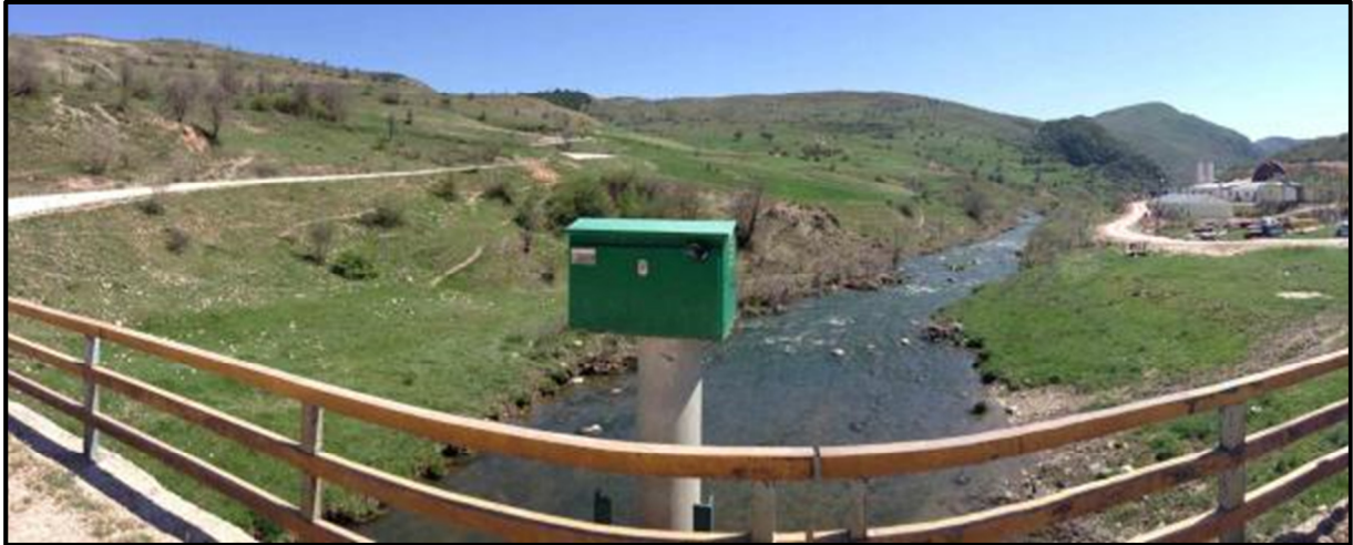
Photograph-6. New Gauging Station
