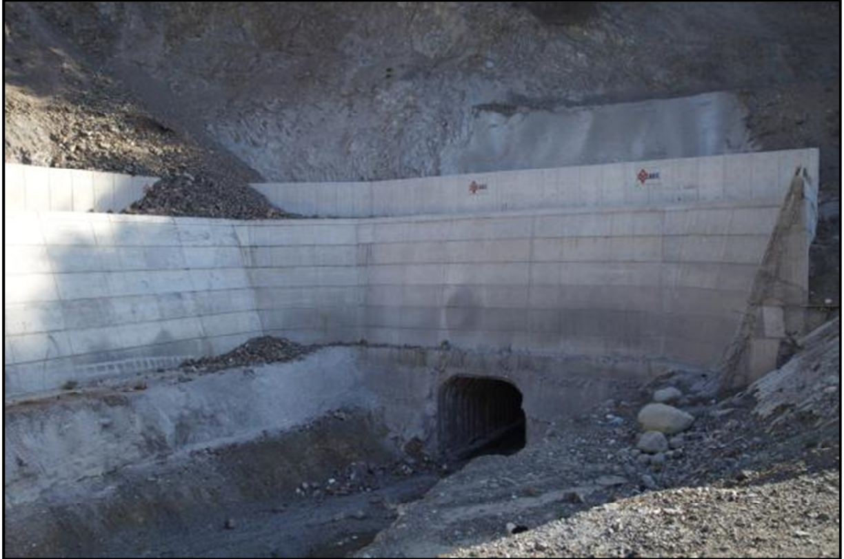
Photograph-10. Kutay HPP Tunnel Entrance
