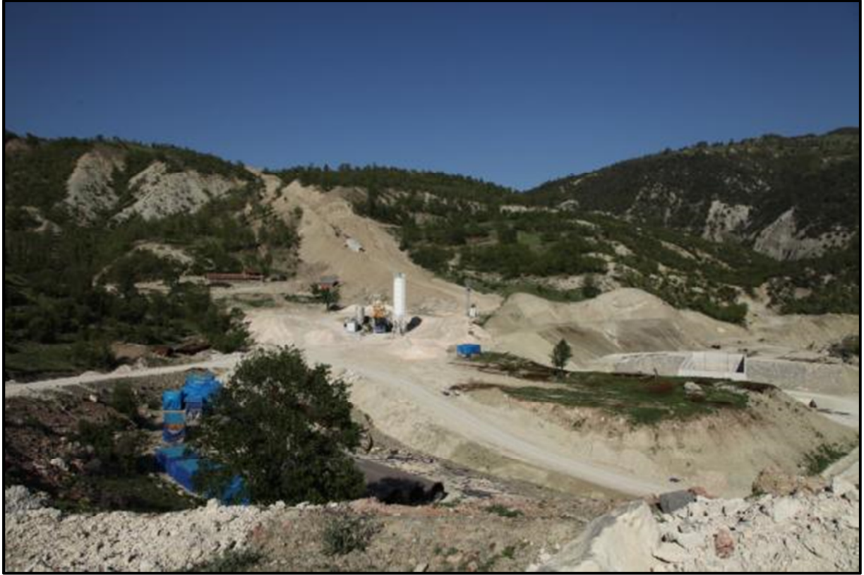
Photograph-9. Çamlıca HPP, Penstock and Powerhouse Construction
